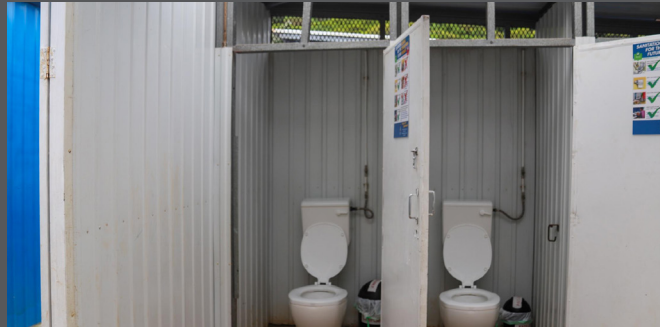
The City's innovative Non-Sewered Sanitation technology project was launched at the Pholani Informal Settlement in La Mercy. These toilets form part of a range of innovative sanitation technologies the City is piloting.
